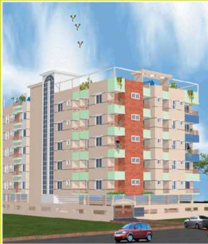
T. A. Abdul hai Garden (6 Storied Residential Building) Nurer Chala, Gulshan, Badda, Dhaka
