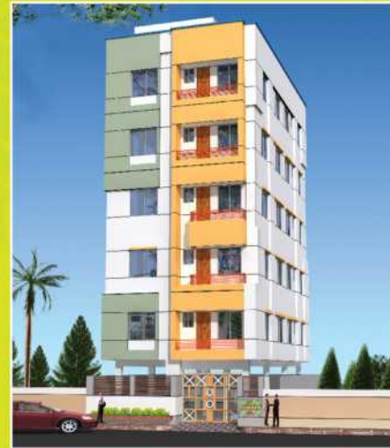
T. A. Jahanara Villa 6 Storied Residential Building Shahjadpur, Progoti Sarani, Gulshan, Dhaka
