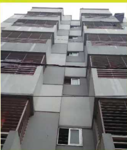
T. A. Rahman Garden (6 Storied Residential Building) Modhubag, Dhaka
